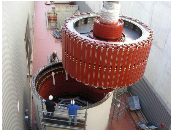
Figure 7.1 – Photo of a turbine undergoing maintenance. The rotor is extracted from the stator in this operation. Source: CNR.
