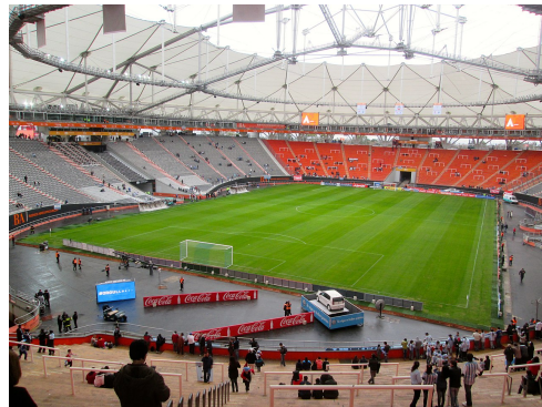
(b) Roof of a stadium in Plata, Argentina (Source: [Pla])
