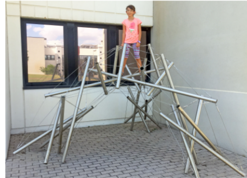
(b) Three-legged tensegrity structure (Source: [Pie+17])
