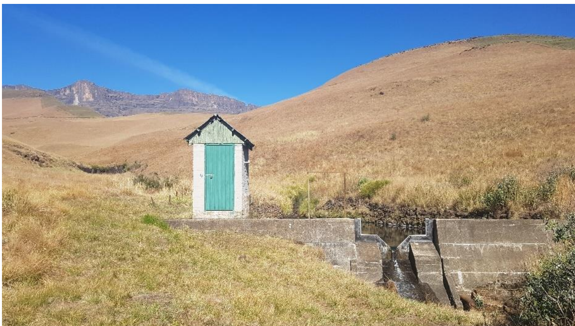
Figure 3.2: Concrete weir and stilling hut, with 90-degree V Notch installed at CP-VI
