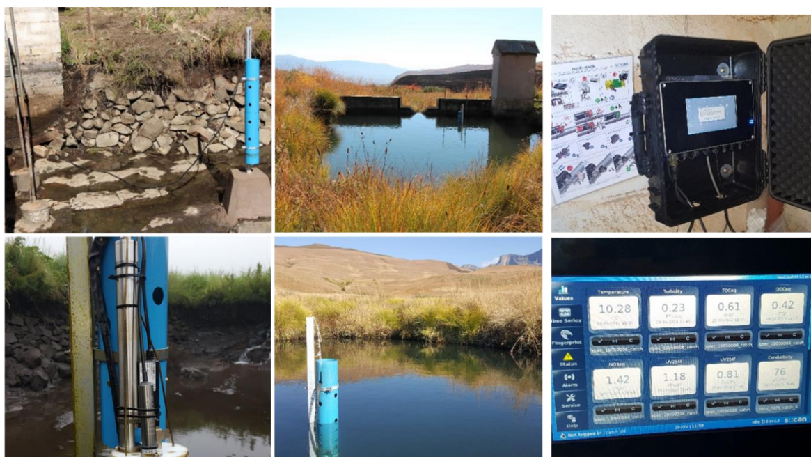
Figure 8.1: The different components of the UV–Vis probes installed at the weir in CP-VI and CP-IX, including the data logger installed in the weir hut
