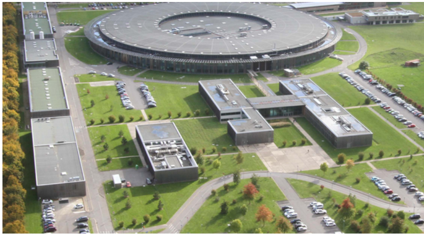
FIGURE 1.3 – Photo du synchrotron Soleil.
