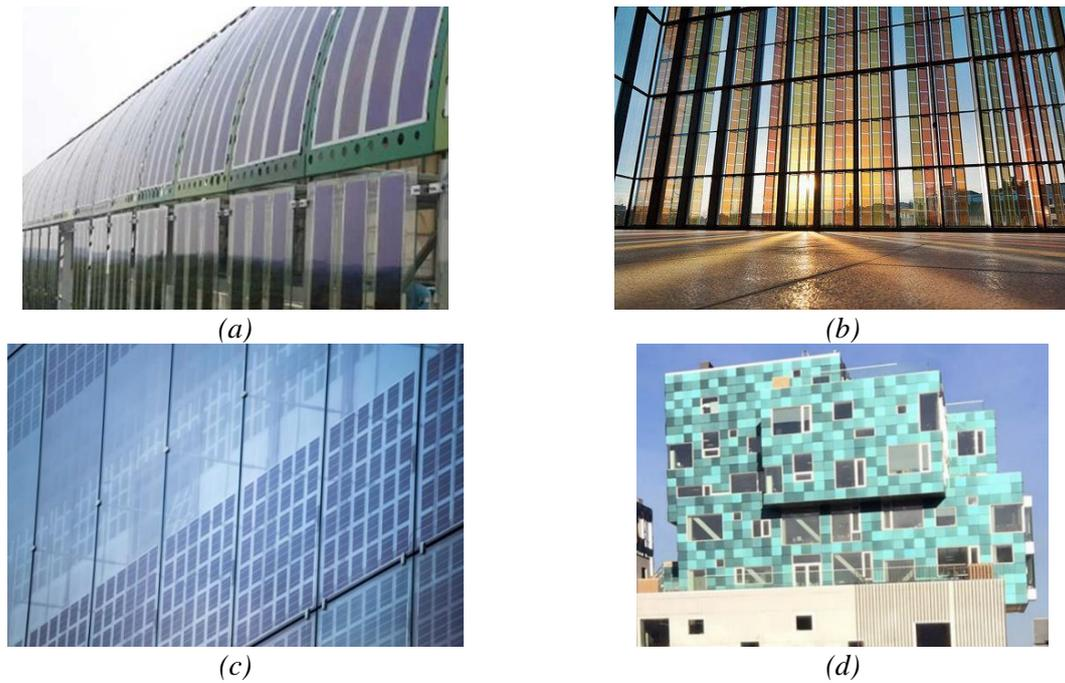
Figure I-5: (a) Flexible PV module ([source: Heliatek](#)) (b) Transparent coloured PV module on the facade of SwissTech Convention Center, EPFL, Switzerland ([source: Solaronix](#)) (c) Semi-transparent PV module on double skin facade ([source: Glassbel](#)) (d) Opaque coloured PV module on the facade of Copenhagen International School ([source: SolarLab](#))
