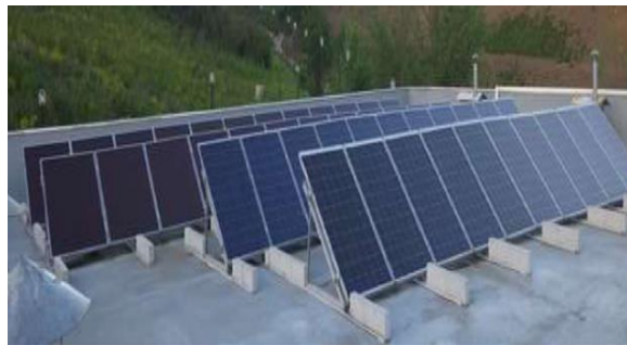
Figure 2-21: Fixed PV system assembly
