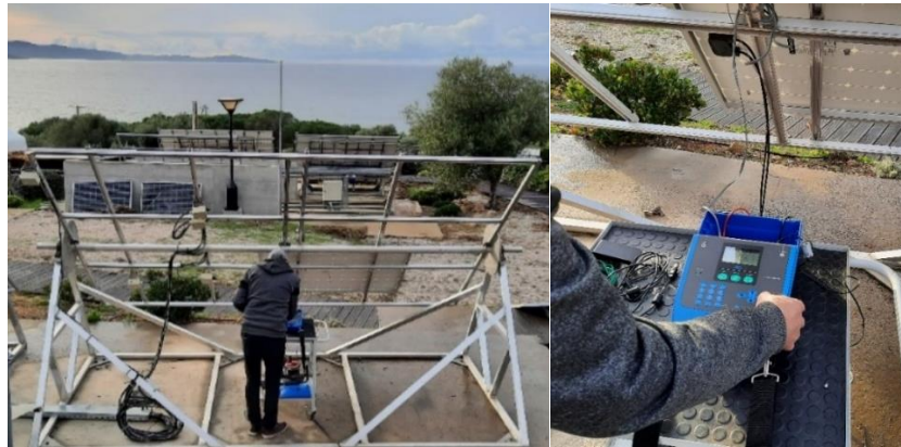
Figure 3-19: I-V tests with the PV modules before installation on the tracker
