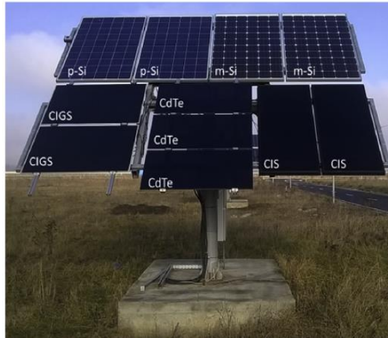
Figure 2-22: Tracking PV system assembly
