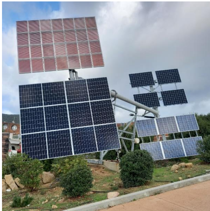
Figure C-1: The PV tracker position during sunrise
