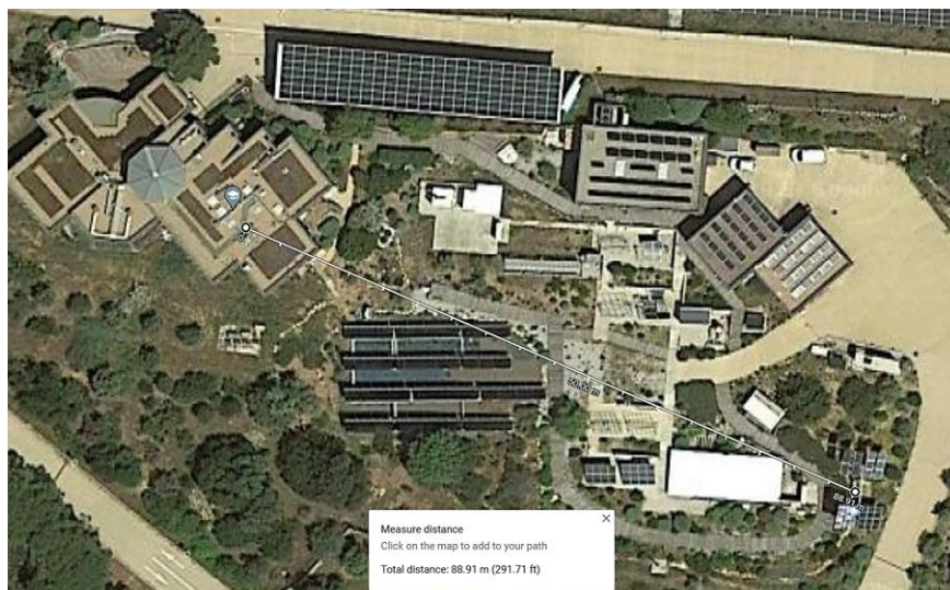
Figure 5-21: Distance between the BNI meter and the HCPV array
