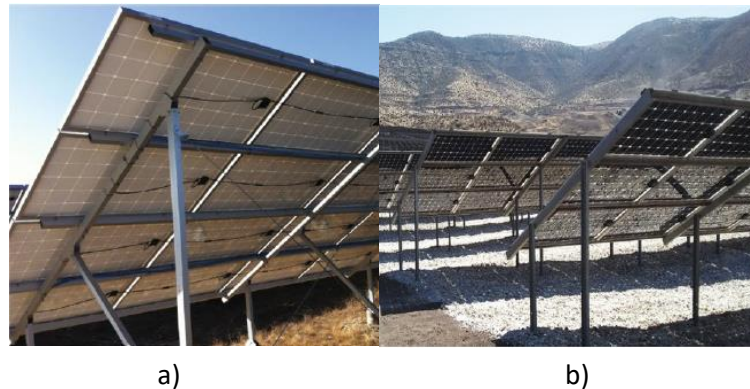
Figure 2-17: Back side of PV modules: a) monofacial; b) bifacial
