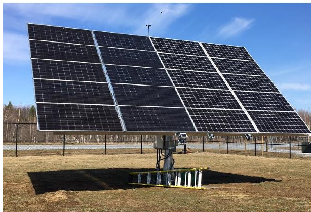
Figure 2-24 – A tracker with 10 monofacial modules (right) and 10 bifacial modules (left). Source: Burnham et al. (2019)
