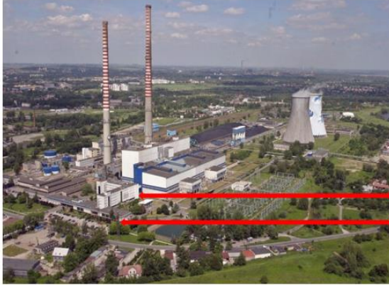
The production building
