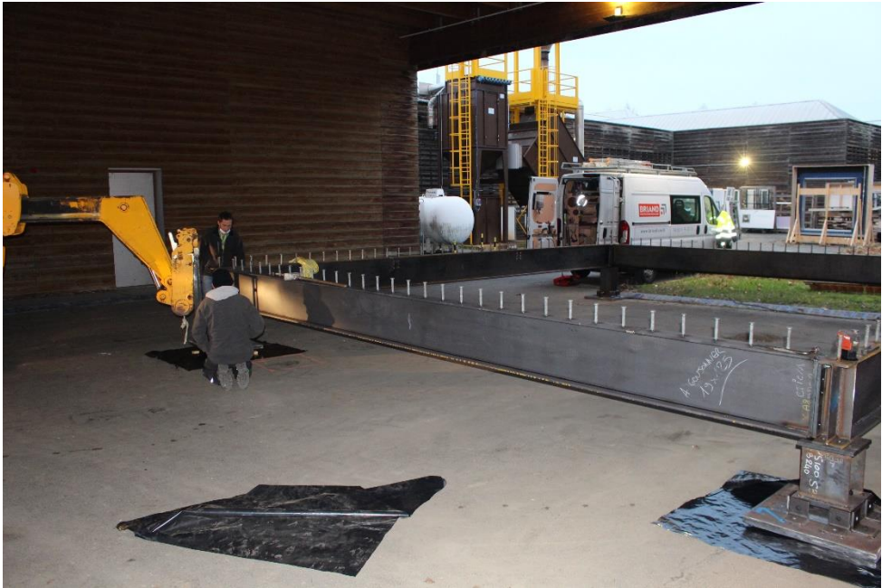
Figure A.6: Shear connectors welded to beams
