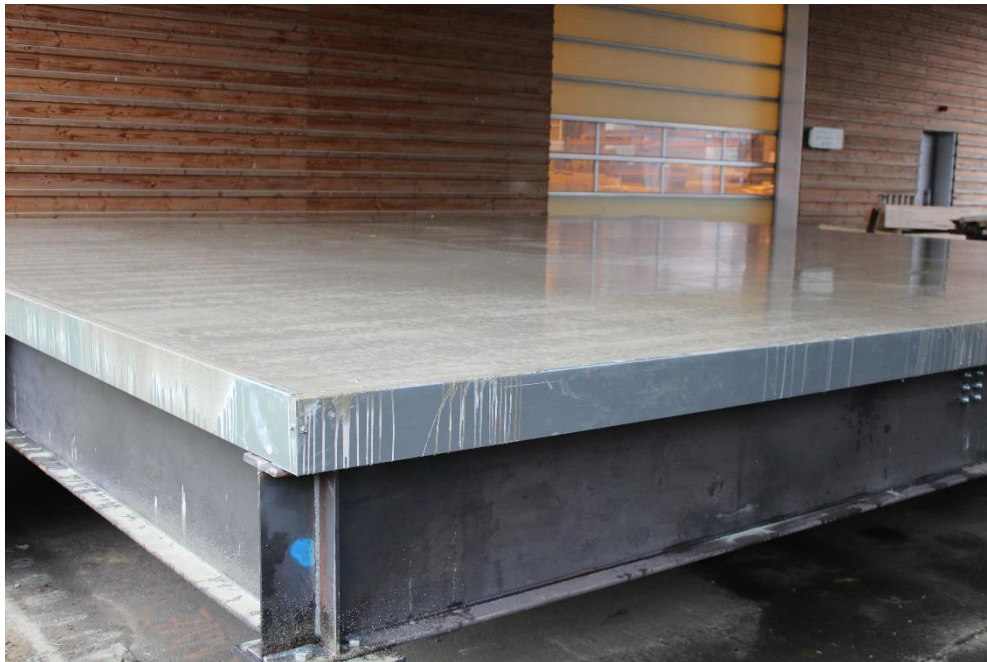
Figure A.8: Floor with composite slab
