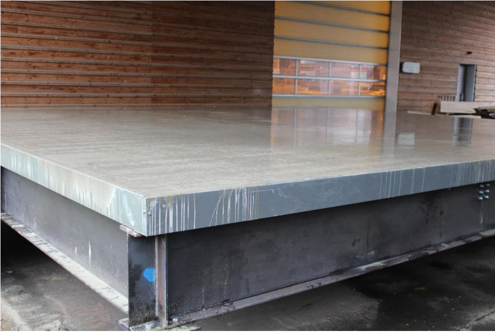
Figure A.8: Floor with composite slab
