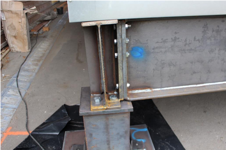
(b) Edges beams
