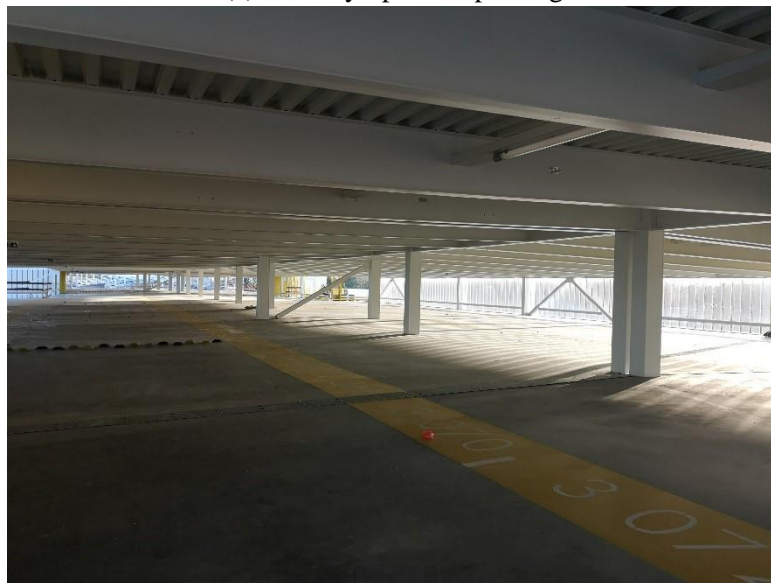
(b) Tested floor area
