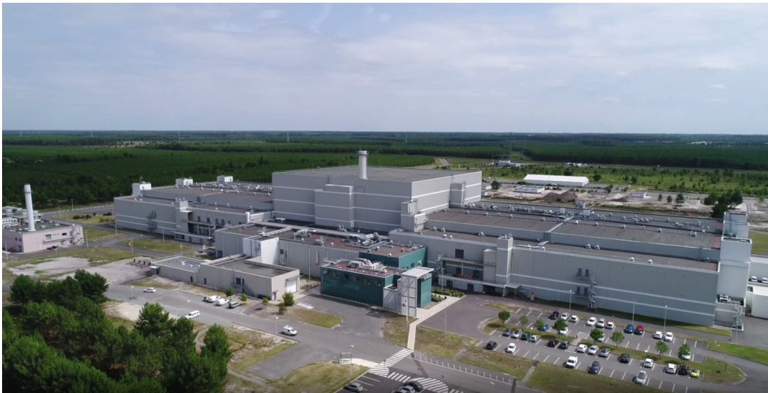
Figure 1.1: Laser Megajoule facility in France [27].
