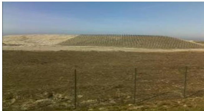
Figure 22. Eco-landscaped merlon at the GPMD
