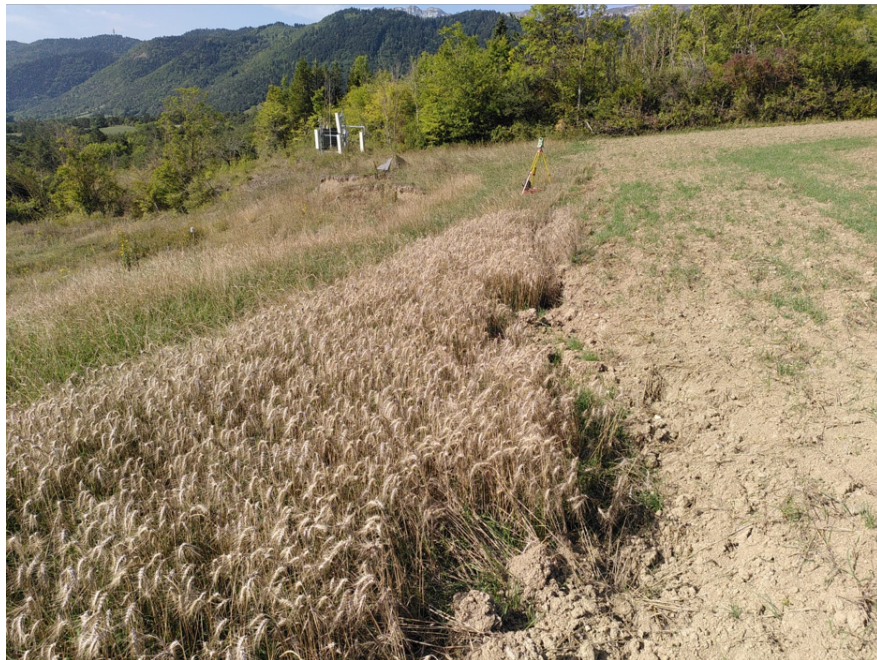
The cultivated field above the landslide is affected every year by the headscarp progression. On the bottom picture, the wheat that was sown before the scarp retrogression could not be harvested.
