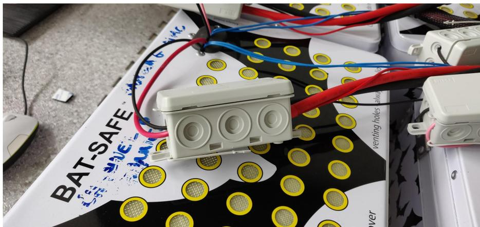
Figure 5.2: Protection boxes for connecting lugs
