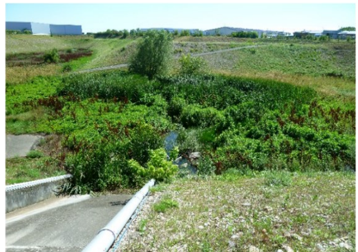
Django Reinhardt bioretention basin, Lyon, France
