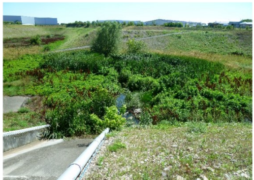
Django Reinhardt bioretention basin, Lyon, France
