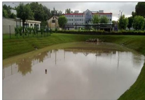
Bioretention basin located at campus INSA, Lyon, France
