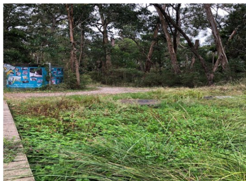
Wicks reserve bioretention basin, Melbourne, Australia
