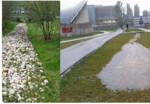
Drainage lawn swale
