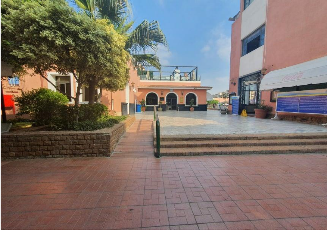
Figure 51: General view of H.S.C and the clubhouse building, Cairo, Egypt
