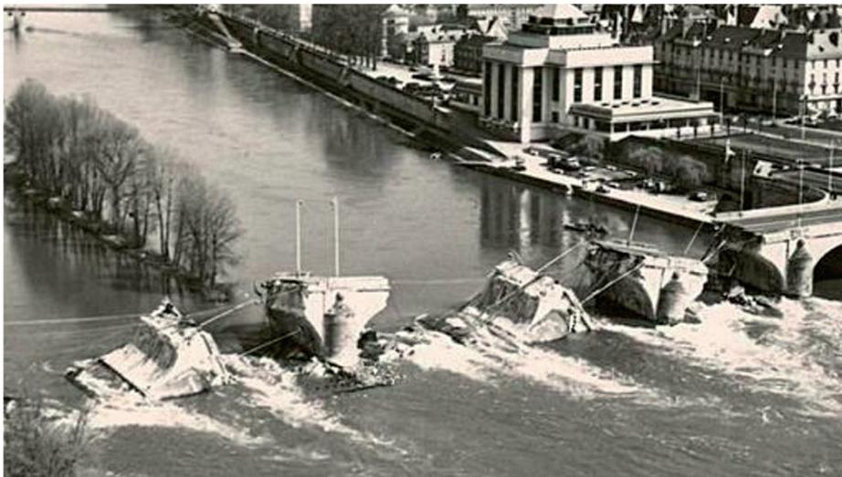
Figure 1-1. Collapse of Wilson Bridge (Tours, France) in 1978 due to general scour; source: Cerema (2019)
