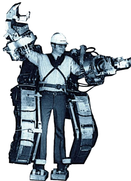
Figure 4. Un des premiers exosquelettes industriels. Hardiman, General Electric, 1965.
