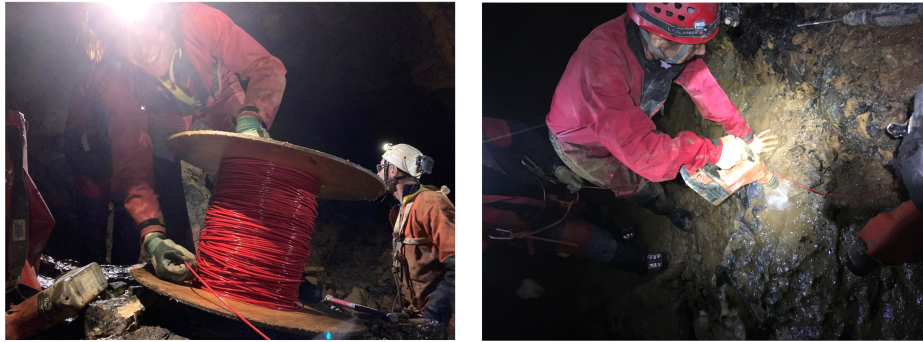
Fig. 2.20 Deployment of the optical fiber cable in the underground conduit.
