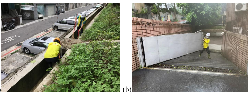
Figure 5-4. Local residents of Dahu area helping (a) clean ditches, and (b) operate floodwalls for a typhoon event on 4 June 2021. (source: Center for Weather Climate and Disaster Research (2021))
