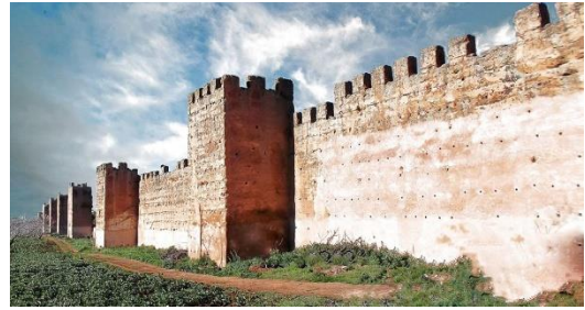
Figure 51 Remparts de Mansourah. Source : (thecasbahpost.com 2023)
