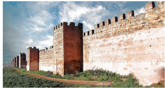
Figure 51 Remparts de Mansourah. Source : (thecasbahpost.com 2023)
