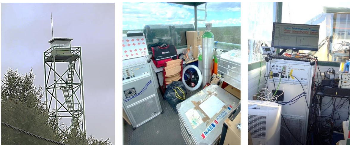
Figure 4.3. Photos showing, from left to right, the room atop of the tower, the installation of the \text{NO}_3^- ToFCIMS and the instrument in its acquisition mode during the ACROSS summer campaign.
