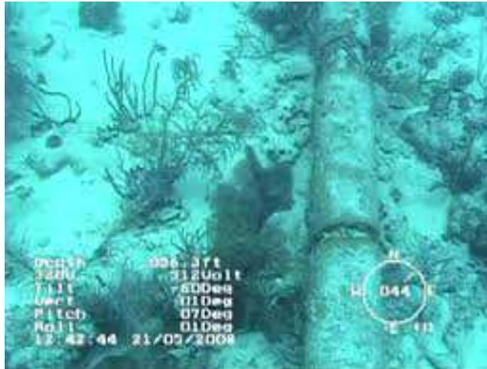
Figure 1.12: An example of pipeline lying on a shallow sea bottom – here, the bottom and the pipe are overgrown due to the presence of sunlight, with edges of the pipeline partially masked, posing challenge to automatic feature detection in the image.
