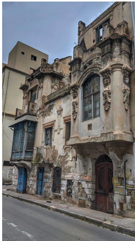
Figure 18. "Villa Yvonne" rue du Luxembourg. (Source: Lost in Tunis, 2020)
