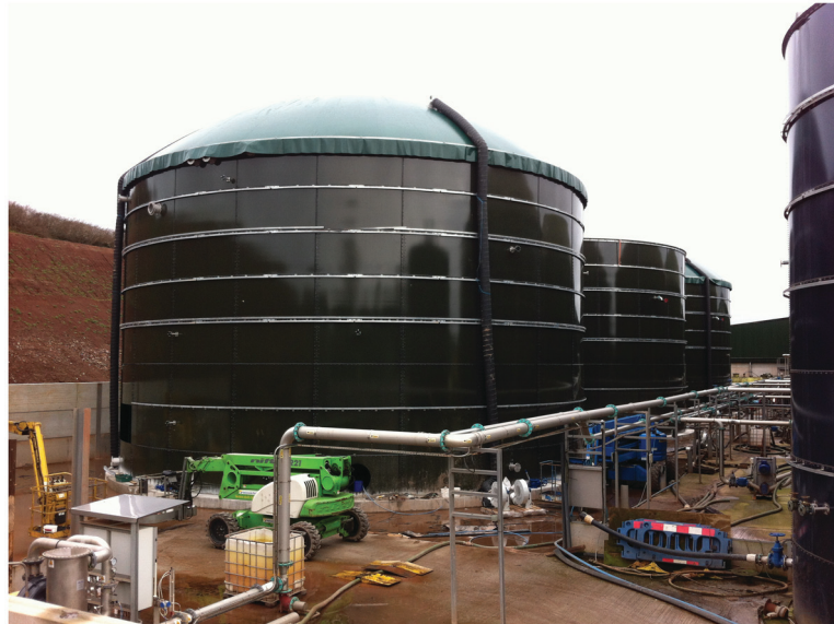
Figure 15. Biogas production plant at the Cannington Cold Stores site. (© 2014, Kirk Group. Used with permission).
