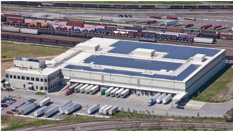
Figure 6. Solar park on the roof of MTC Logistics' cold store at the Port of Baltimore. (© 2011, HelioSage. Used with permission)
