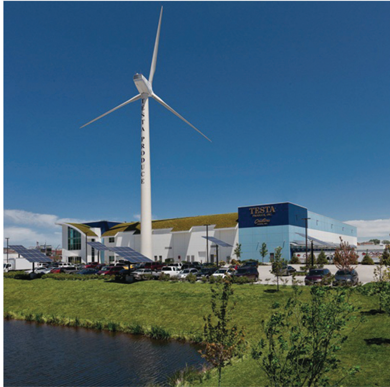
Figure 10. Testa Produce's LEED Platinum-certified refrigerated food distribution facility in Chicago, featuring a 750 kW wind turbine. (© 2013, Epstein. Used with permission)
