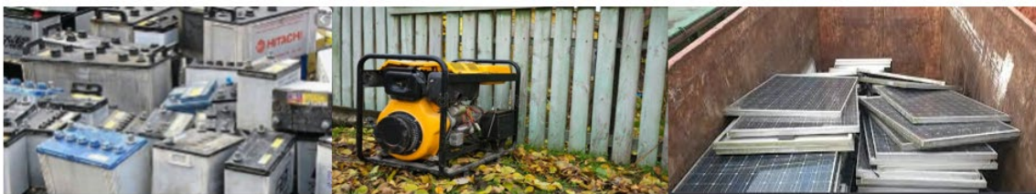
Figure 1.8 – Legacy batteries, generator, and PV panels [12]
