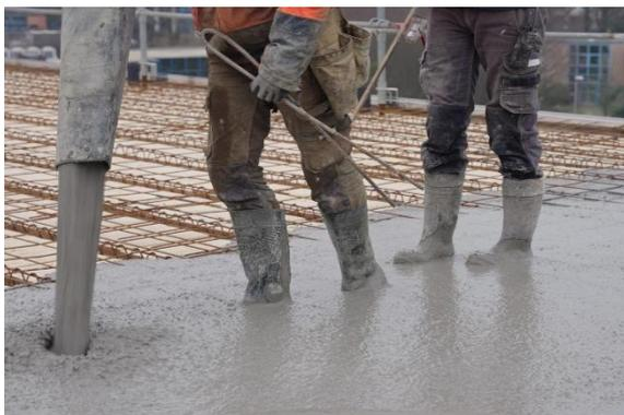
d. Casting of concrete panel
