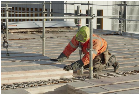
b. Installation of CLT panels
