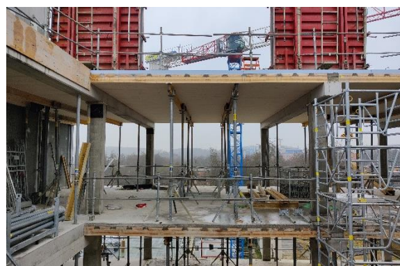
e. HOB OA floor system after concrete casting
