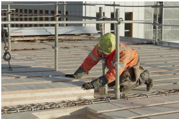
b. Installation of CLT panels
