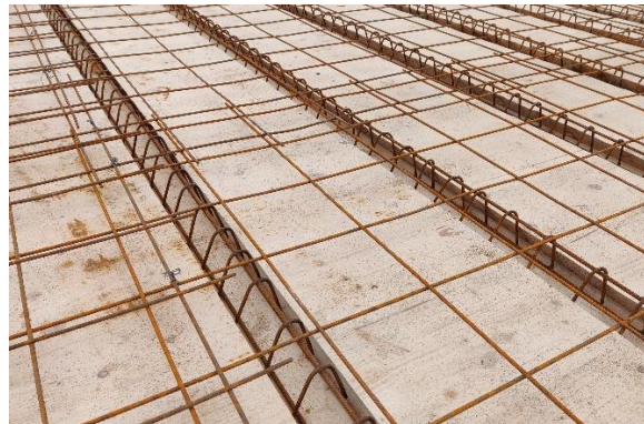
c. Installation of V-shape rebar cages and steel meshes.
