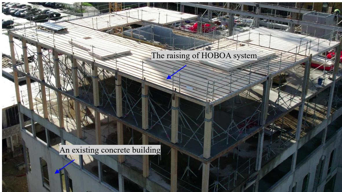
a. An existing concrete building with the application of HOB OA floor system
