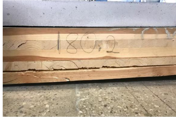
c. Failure of specimen F2
