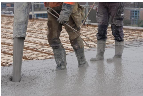
d. Casting of concrete panel
