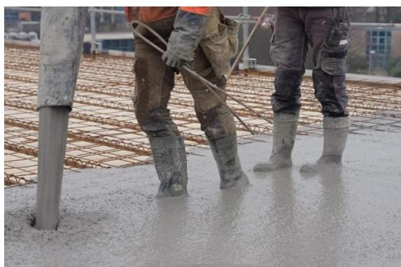
d. Casting of concrete panel
