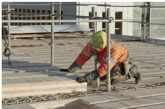
b. Installation of CLT panels
