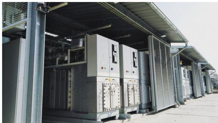
Figure 1-3. Schematic of the current world's largest SOEC system within the MultiPLHY hydrogen project by Sunfire (14).
