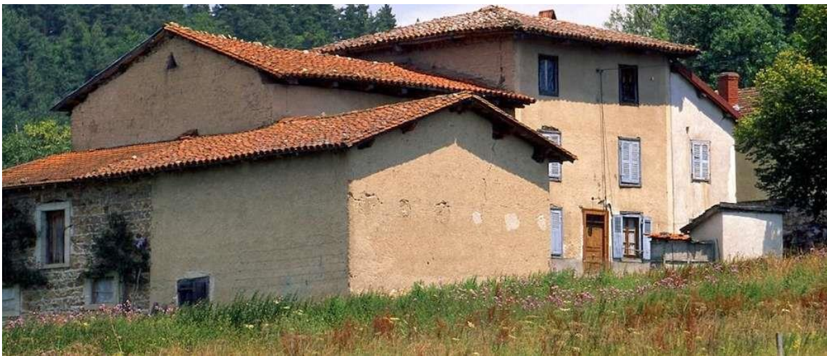
Figure 1.4: An example of a traditional rammed earth building located Marsac-en-Livradois, Puy-de-Dôme, France
