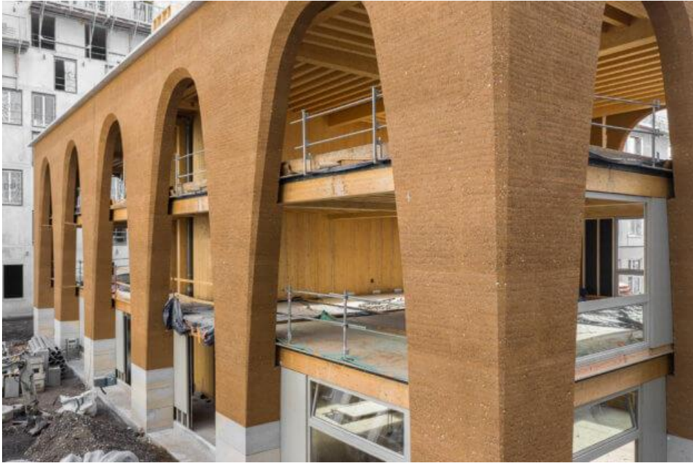
Figure 3.1: Modern rammed earth building at Confluence, Lyon.
