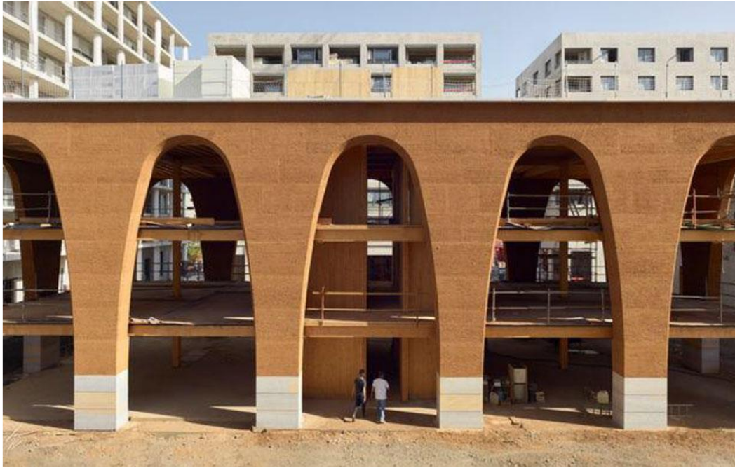
Figure 1.5: Modern architectural rammed earth building Confluence in Lyon (source: Clement Vergely architects/Fabrice Fouillet).
