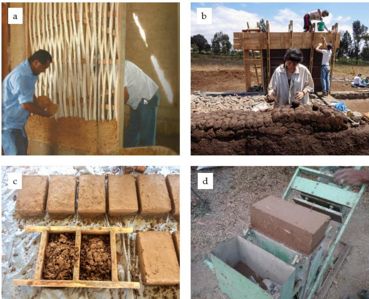
Figure 1.2: (a) Wattle and daub [26], (b) Construction of a cob wall by stacking mud balls [10], (c) Adobe (source: Archaeology Southwest), (d) Compressed earth blocks [27].
