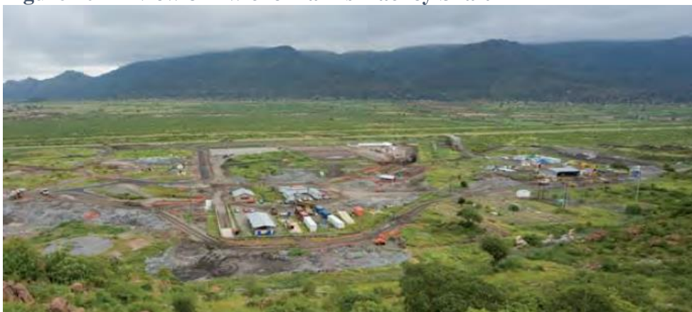
Figure 20 - A view of Twickenham's Hackey Shaft
