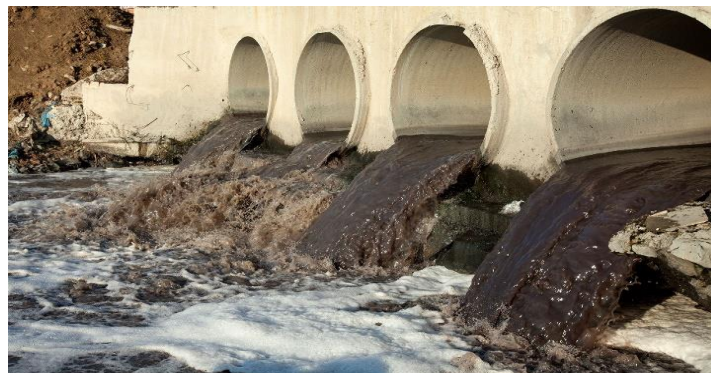
Figure 3 Raw sewage discharge in the rivers 3
