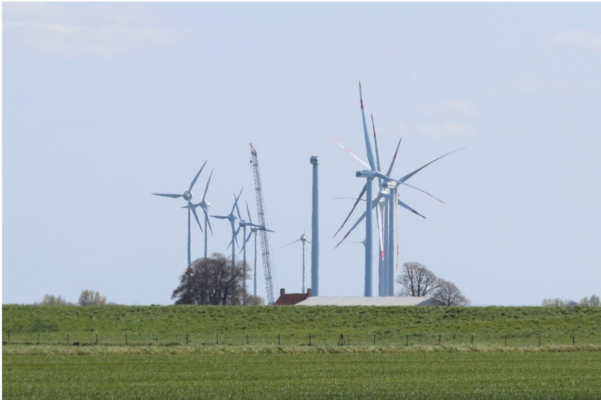
Figure 1.3: “Repowering” of a wind farm: nine old small wind turbines (left; 0.5 MW, rotor diameter 40 m, ground clearance 45 m) are replaced by six new large turbines (right; 3.4 MW, rotor diameter 114 m, ground clearance 36 m; Dutch-German border, study area Groningen). Photo: T. Schaub.
