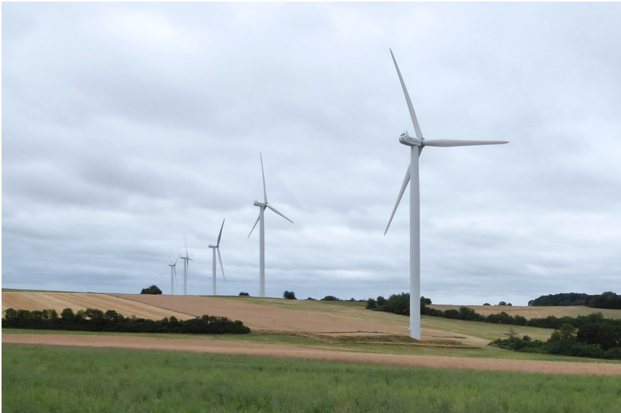
Figure 1.1: Wind farm in an agricultural landscape (study area Alsace/FR). Photo: T. Schaub.
