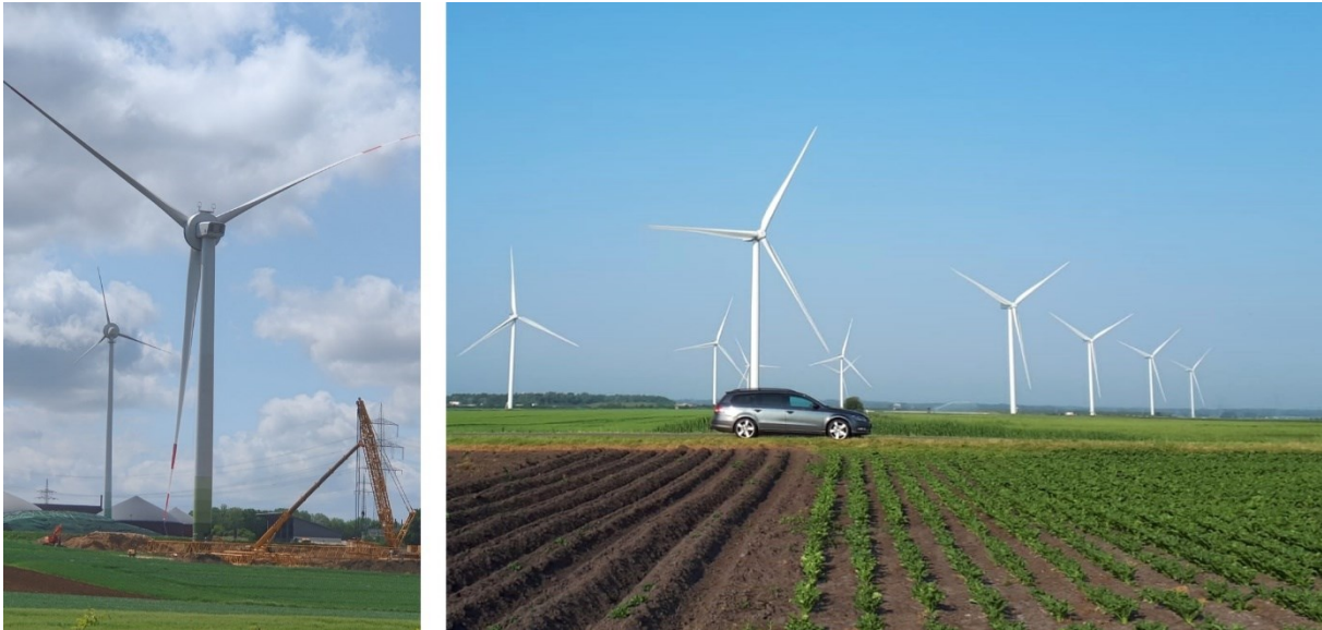
Figure 6.2: Examples of recently installed wind turbines with particularly low ground clearance. Left: Ground clearance 11 m, diameter 138 m, 4.2 MW, installed in 2023 (in comparison to older turbine with higher ground clearance [45 m] and smaller rotor diameter [40 m; 0.5 MW] in the background). North Rhine-Westphalia, Germany. Right: Ground clearance 18.5 m, diameter 131 m, 3.6 MW, installed in 2022. Drenthe, the Netherlands. Photos: H. Illner, H. J. Ottens.
