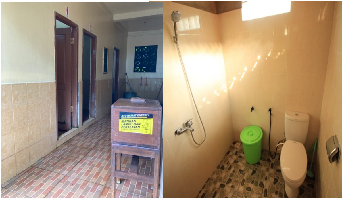
Figure 52 Upgrade of Nglanggeran village's lavatories with the support of the local government
