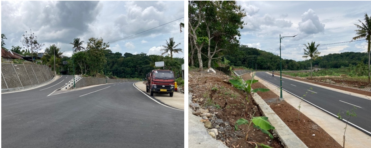
Figure 100 Construction of the main road around the village of Nglanggeran
