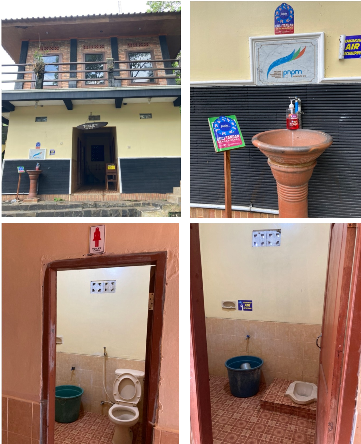
Figure 47 Facilities and infrastructure (toilets and rooms) the result of the cooperation of various parties
