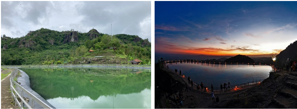
Figure 50 Government investment in dams infrastructure around Nglanggeran village
