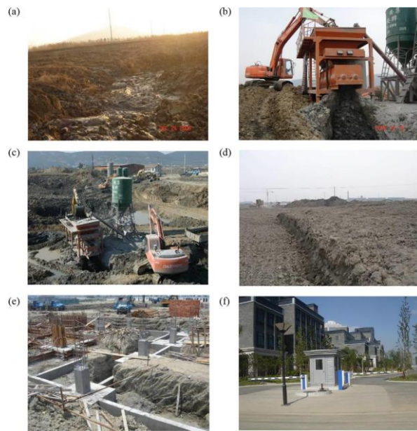
Figure 1-9 Using solidified dredged sediments as fill materials at Wuxi, China: (a) dredged sediments before treatment; (b) used machine for solidification; (c) the large-scale working field for treatment of sediments; (d) backfilling with treated sediments; (e) construction activities on the backfilled treated sediments; (f) the project is completed and put into use [79].
