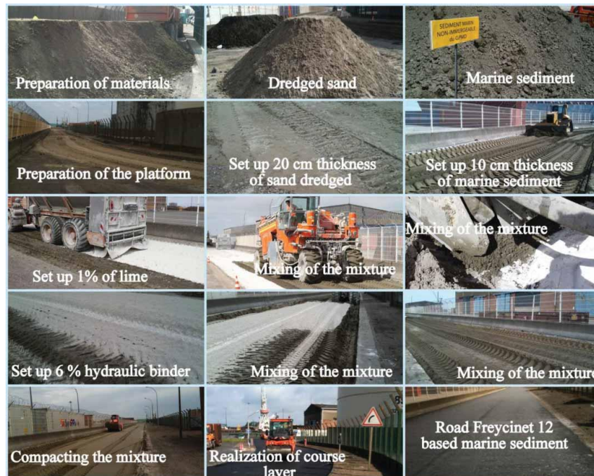
Figure 1-8 Build Freycinet 12 experimental road with solidified sediments at Dunkirk, France [53].
