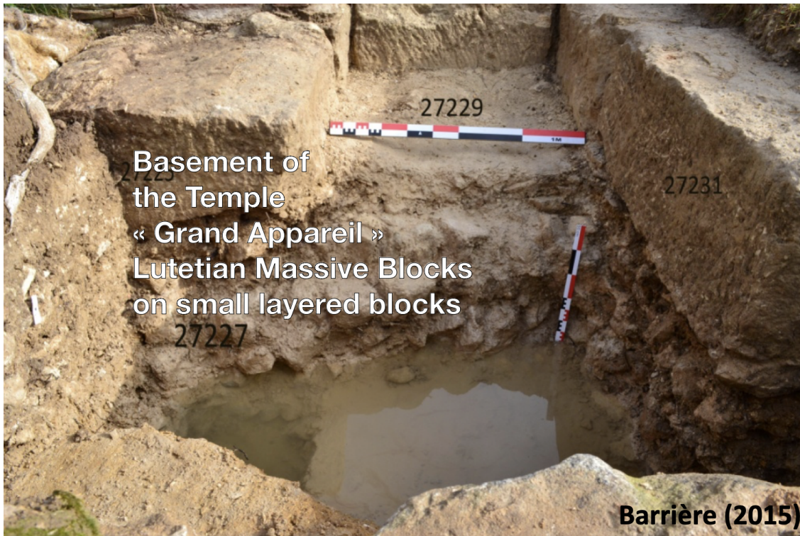
Figure 2.18: Basement of the temple in contact with groundwater (Barrière, 2015).
