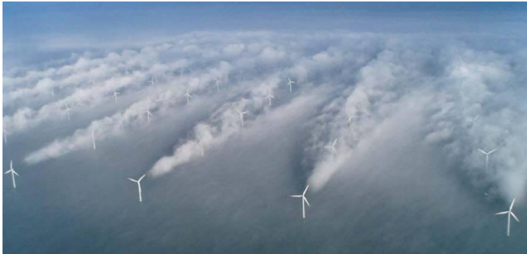
Figure 1.7: Photography of the Horns Rev 1 wind farm. Photography taken by C. Steiness for Vattenfall. Taken from Hasager et al. (2013).
