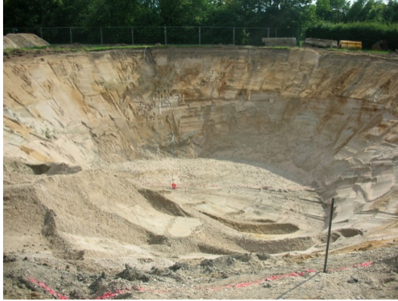
FIGURE 1.28 – Excavation du PTES de Eggenstein-Leopoldshafen[40].
