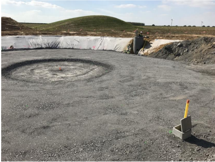
Figure 3-11: Position of the inclinometer.
