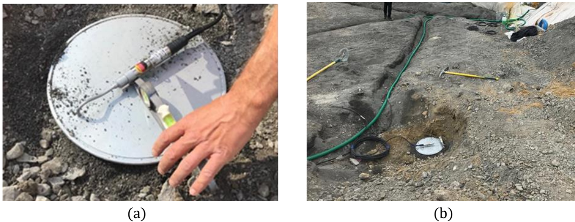
Figure 3-7: (a) EPC installed at the top of the RIs with an equivalent diameter, (b) wiring to the acquisition units.
