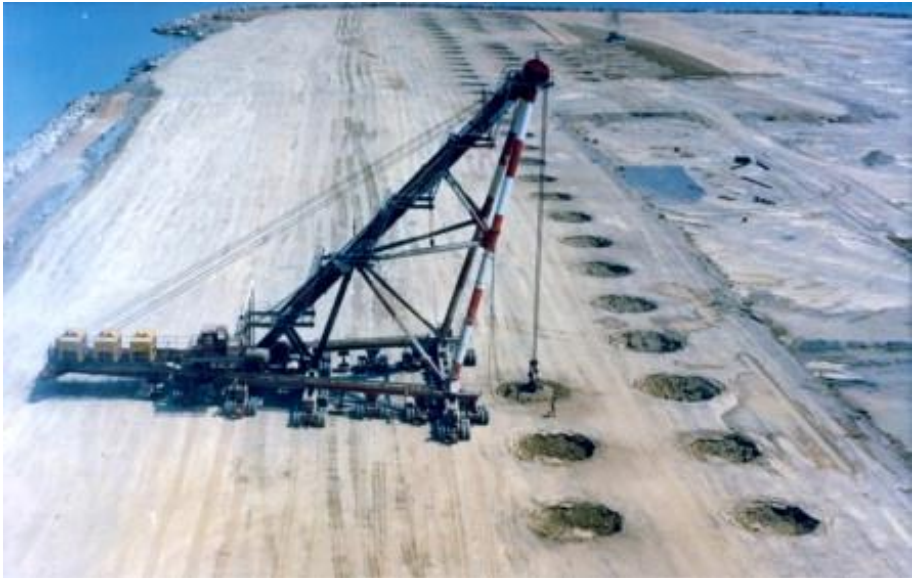
Figure 2-4: Menard's "Giga" compactor drops a 200-ton weigh (Nicholson, 2014).
