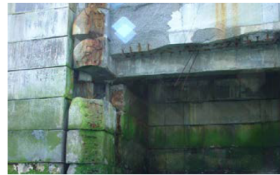
Figure 3.7: (Left) Picture of the WEC of Mutriku after the storm (Right) Picture of a damaged chamber of the WEC
