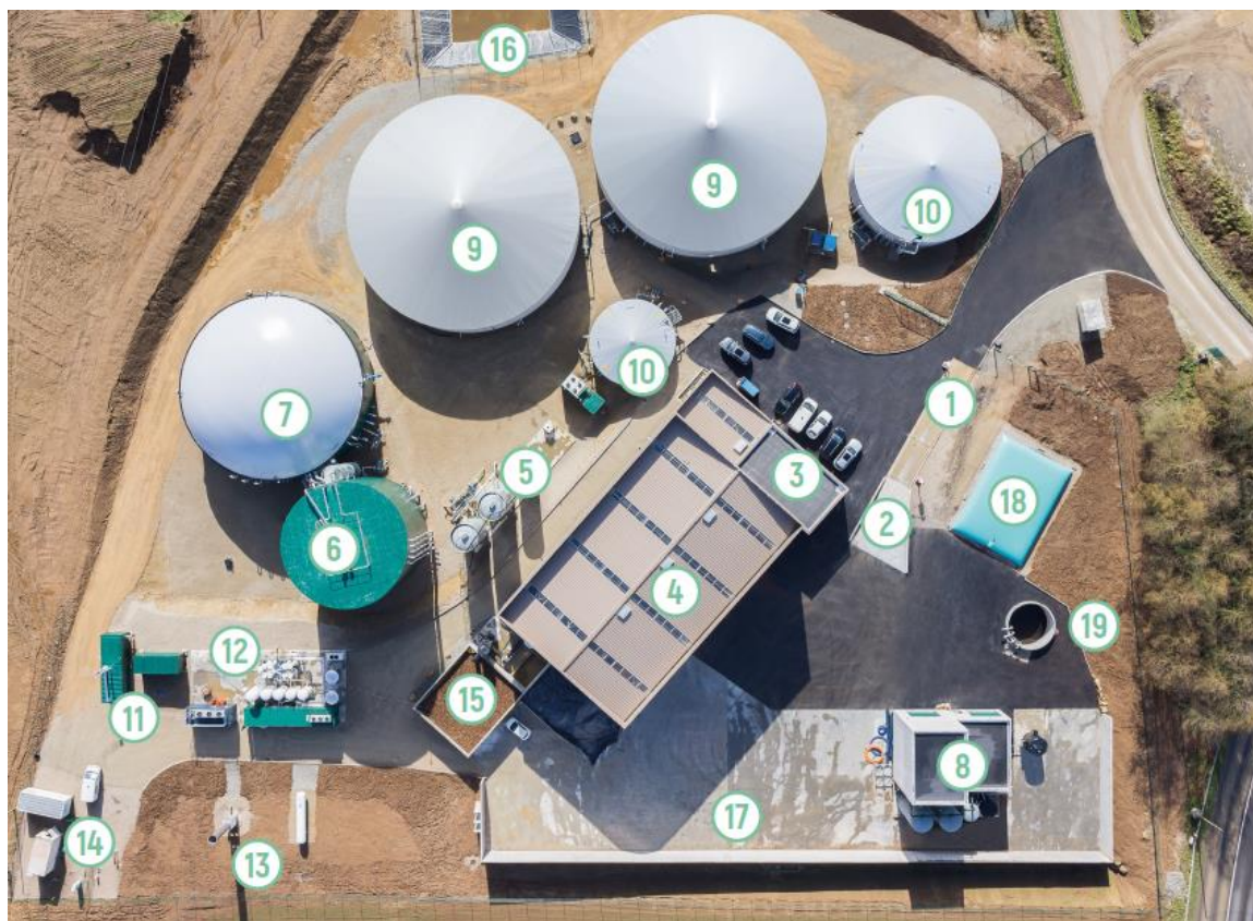
Figure 13 Example of a biomethane plant in France - Source: Engie BiOZ
