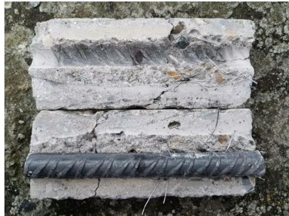
Figure 212 : bottom front bar of G3-07 sample after 30 cycles of wetting-drying cycles
