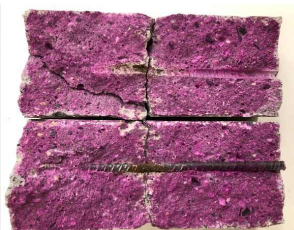
Figure 117 : Carbonation along bottom bar of ref 3 sample
