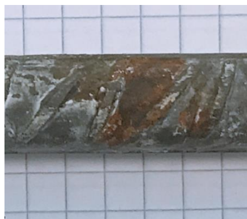
Figure 204 : Zoom of the corrosion at the location of the artificial crack after 4 cycles (top back bar of G3-10 specimen)
