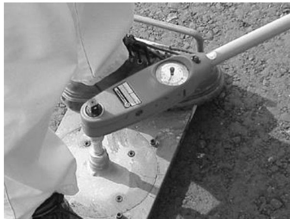
Figure 1.8: Torque bond test device in-situ (Attia, 2020)
