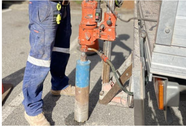
Figure 1.7: Pavement coring (source : (Liquidlabswa, n.d.))
