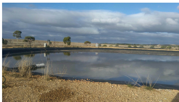
Figure 2.18 – Anaerobic pond upstream Peterborough HRAP
