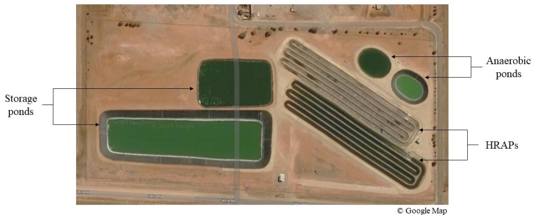
Figure 1.6 – Aerial view of Peterborough wastewater treatment site
