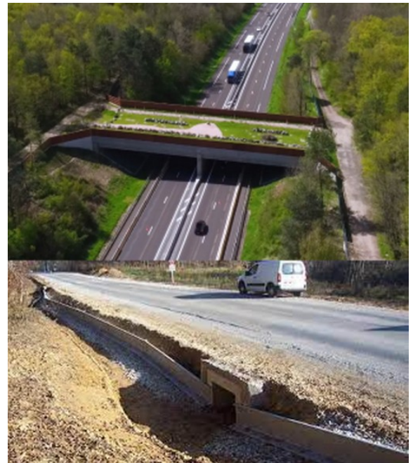
Fig. 2: Example of wildlife crossing structures: the Varennes overpass on highway A89, Puy-de-Dôme, France (top) and an amphibian underpass on road D14 (bottom, located in Doubs, France).
